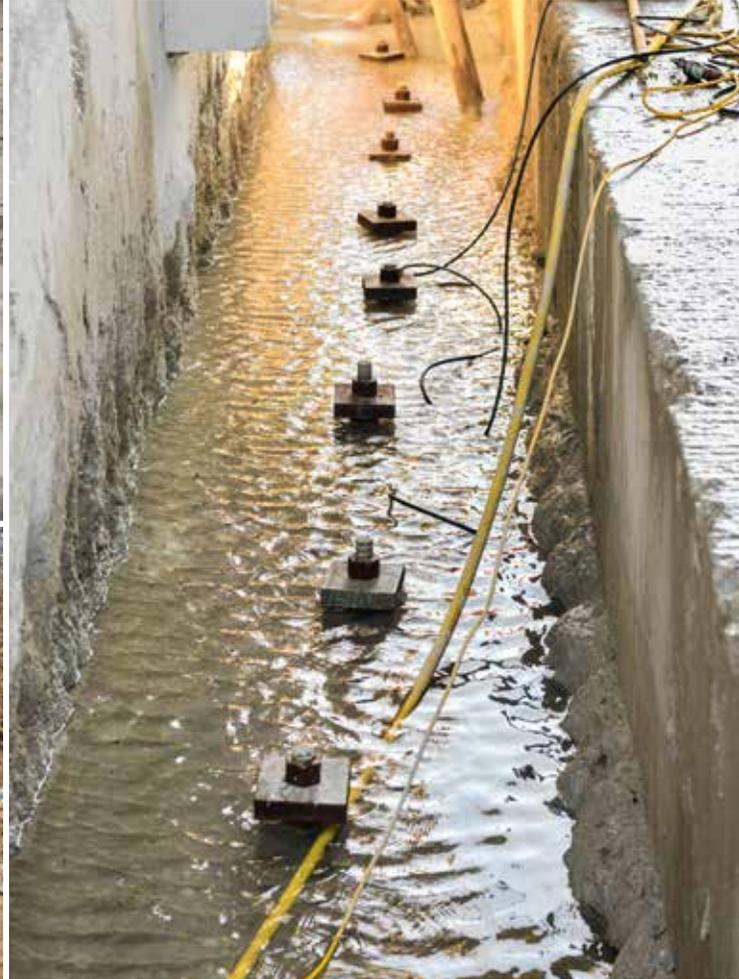
This project also includes the existing Weidenbach railway bridge in the Gaenserndorf-Weikendorf section. The bridge had to be extensively reinforced and stabilized using a *GEWI® Plus* Micropile foundation.
