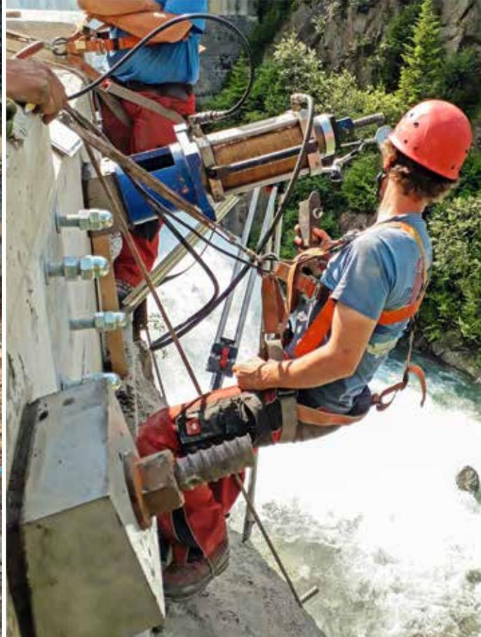
Safety cables, personal protective equipment for the personnel and special equipment for drilling were used during the work.
