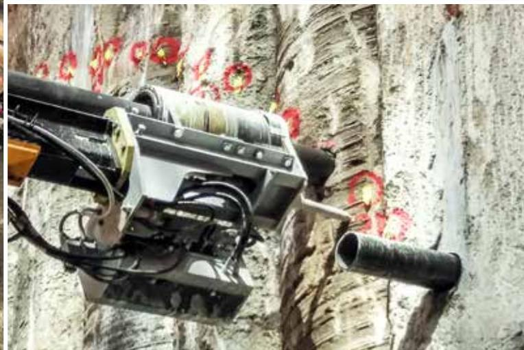
Four stations are being excavated using the New Austrian Tunneling Method (NATM): Oakwood, Avenue, Laird and Leaside. For these stations, DSI Underground Austria has been awarded a supply contract for a self-drilling pipe umbrella support system.
