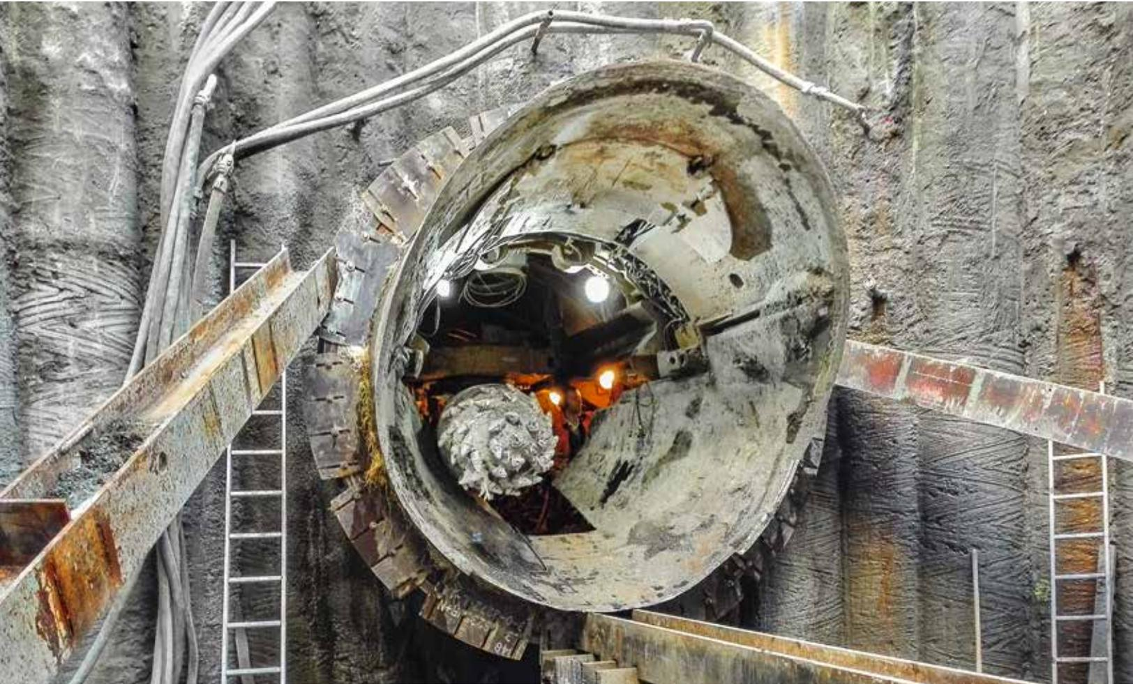
The 35km long section between Dortmund and Bottrop is being built by Wayss & Freytag. The tube advancement was carried out using 9 full section tunnel boring machines (TBMs) and one road header. In total, approx. 15,000 reinforced concrete tubes were pressed in for the construction of the sewer canal. 130 excavations that were up to 40m deep had to be realized as starting or end shafts for the TBMs.
