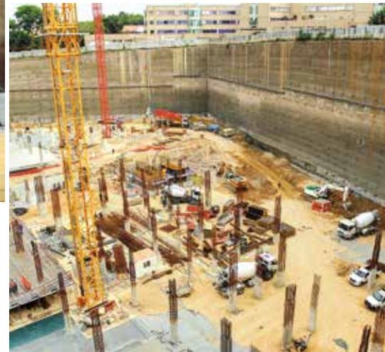
The 24,435m<sup>2</sup> excavation represented a major challenge to all parties involved due to its size and to the work that had to be completed within 12 months. First, the existing buildings occupying the site had to be demolished. The last part of the construction site could only be vacated 4 months after commencing the project.
