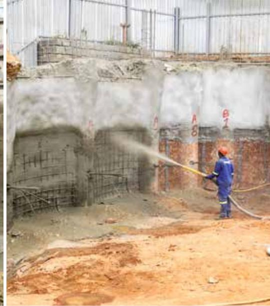
In the first phase, the existing boundary walls with the Balalaika and Protea Hotels had to be stabilized. The second and final phase included the excavation and lateral support to the new proposed basement layout, including the demolition and removal of the existing 4-basement parking garage.
