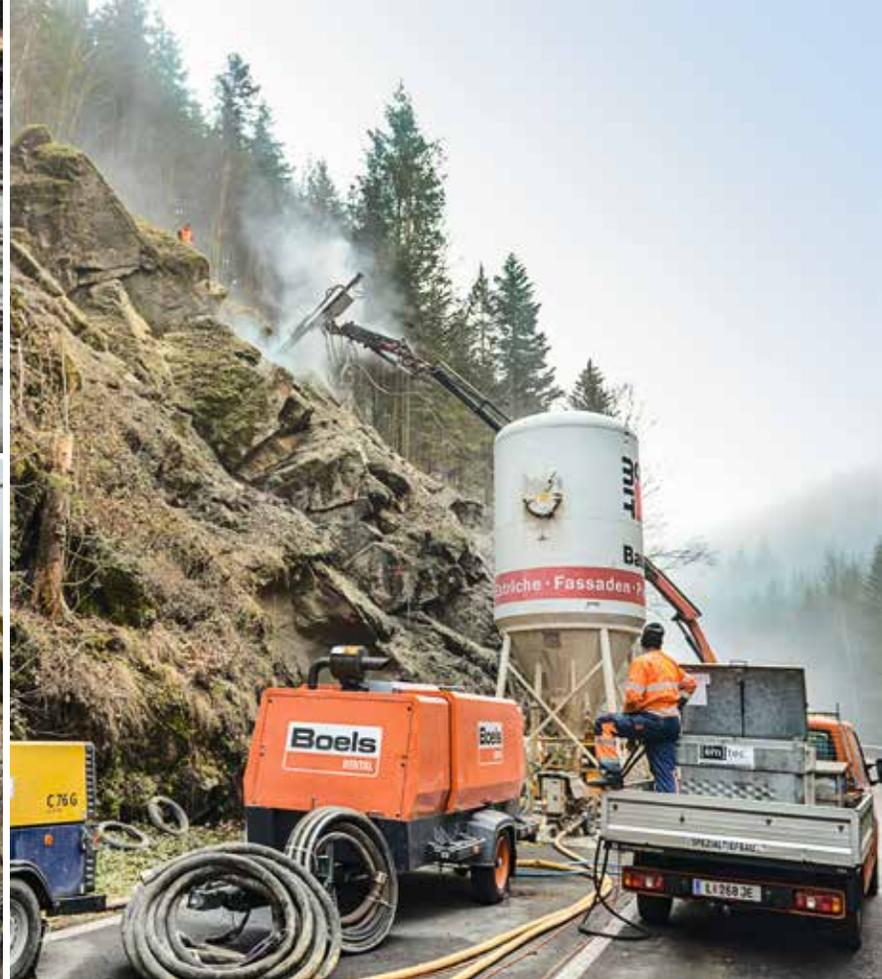
In order to permit a partial reopening of the road, immediate steps were required. The rock face was stabilized from the road using a crane mount from which approx. 750m of boreholes and rock anchors had to be installed. Furthermore, the partly fractured rock was stabilized using 1,200m<sup>2</sup> of rock mesh.
