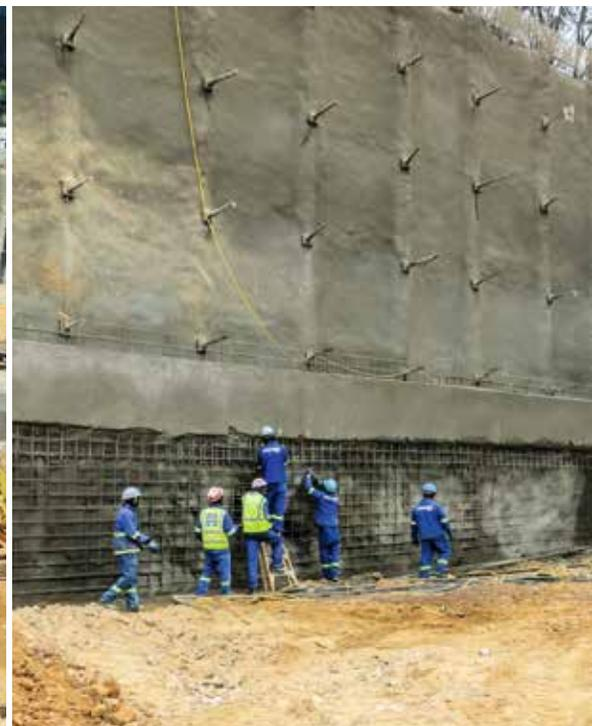
The highly unpredictable geology represented a significant challenge. The excavation support design had to be altered to suit the changing rock levels in the course of the project. The anchor design was only concluded after the soldier pile installation along the complete excavation had been carried out.
