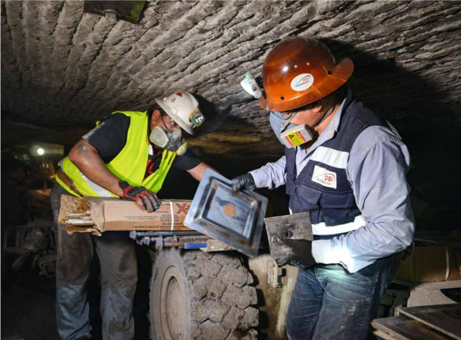
The anchor systems are installed together with 23mm x 760mm FASLOC® Polyester Resin Cartridges. The cartridges ensure an immediate, high load-bearing capacity of the anchors.
