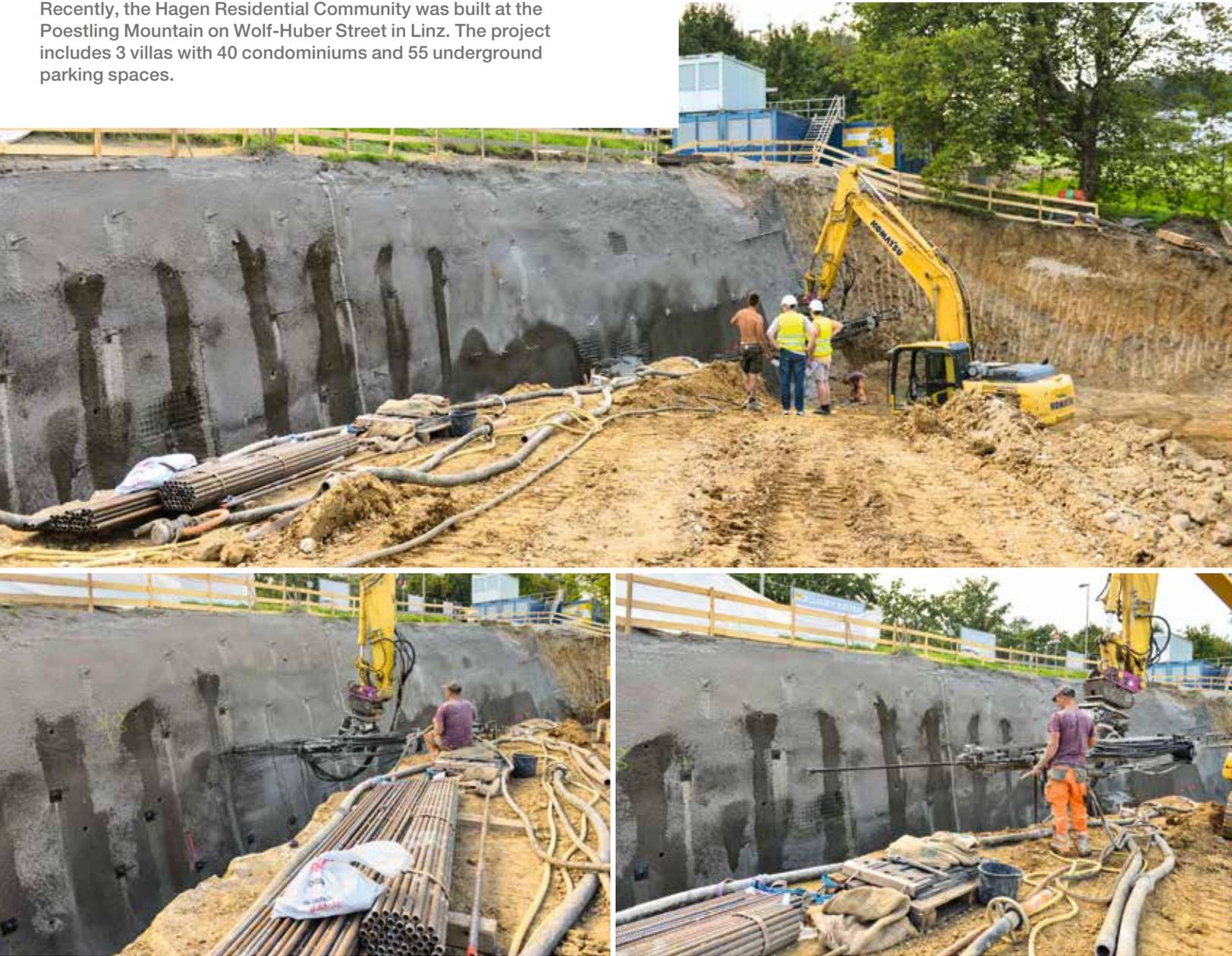
Since the excavation borders a local street, the necessary steep embankment was stabilized by an anchor wall covered in shotcrete. To ensure a fast and safe installation of the anchors, the HABAU Hoch- und Tiefbaugesellschaft m.b.H. company, Austria decided to use self-drilling hollow bar anchors.
