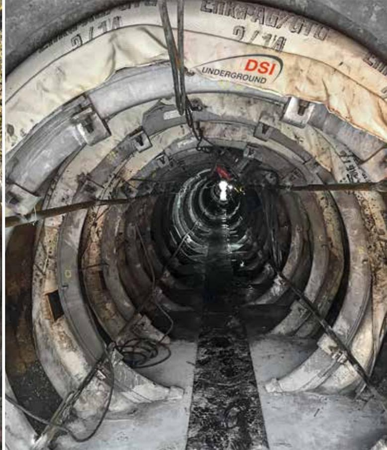
During construction work, traffic disruption on the RN 47 road had to be kept to a minimum. Repair work was carried out inside the tube using a protection cage. The sediment carrying water was pumped off to permit installation of ground support.
